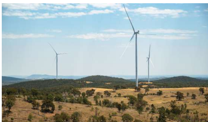
MacIntyre Wind Farm. Image Courtesy: ACCIONA Energia.
